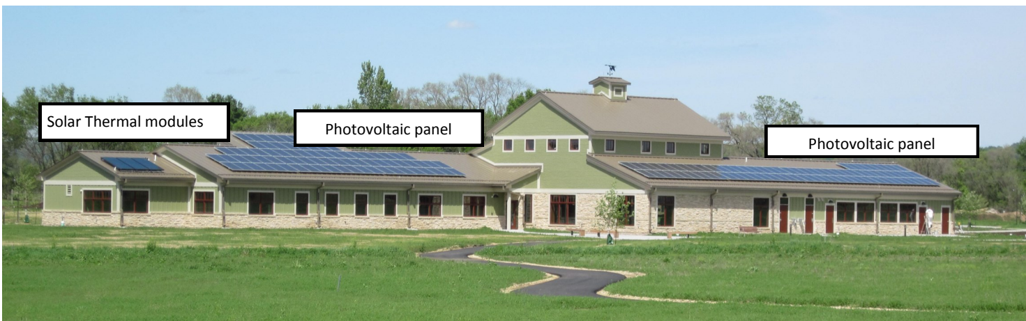
Three solar thermal modules can be seen on the back of the new visitor center . The solar thermal panels utilize sunlight to heat water for the restrooms and sinks. To the right of these solar thermal modules, 156 photovoltaic modules form two panels that transform sunlight into electricity.
